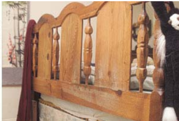
Mold growing on a wooden headboard in a room with high humidity.
